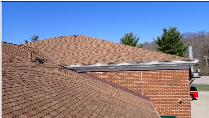
Overview of roof
