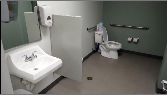
Overview of washrooms
