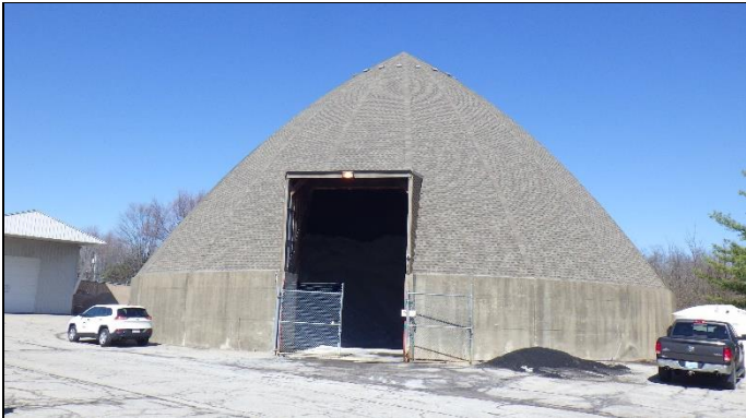
Overview of dome
