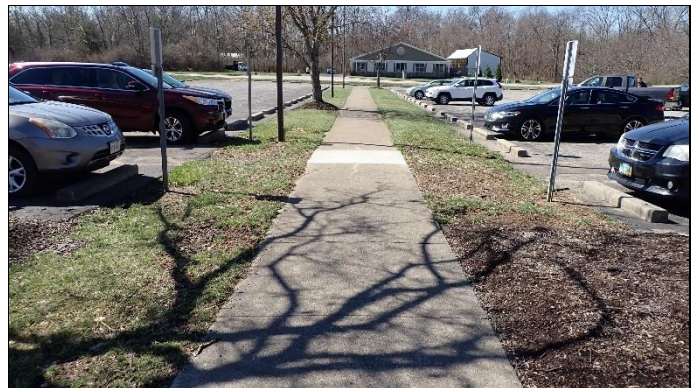
Overview of concrete walkway
