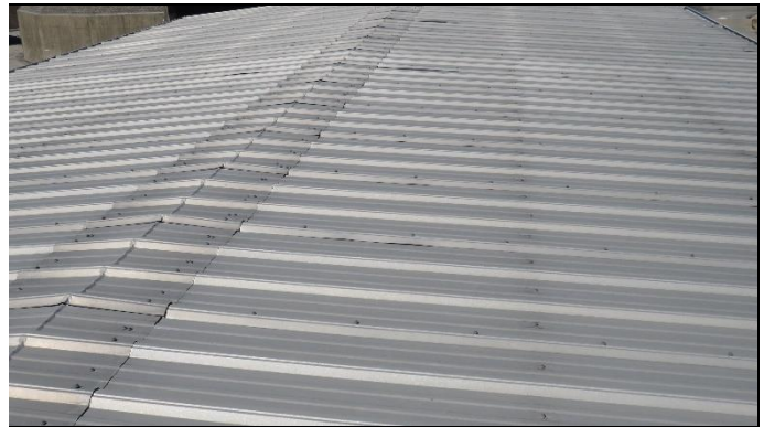
Overview of roof
