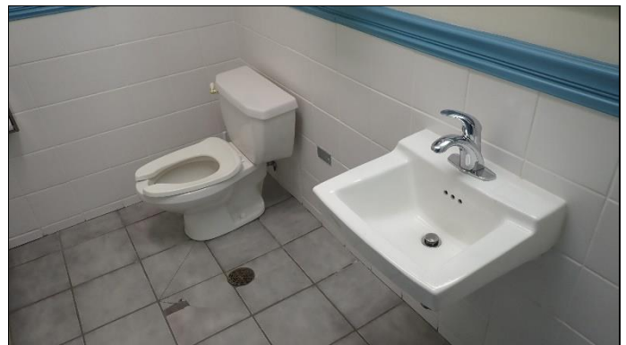
Overview of washrooms
