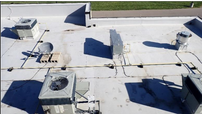
Overview of roof
