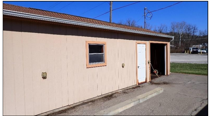
Overview of outbuilding
