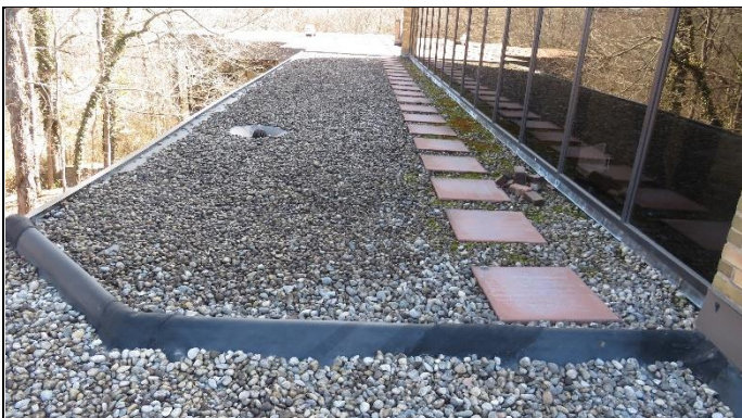
Overview of roof
