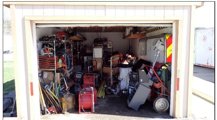
Overview of outbuilding
