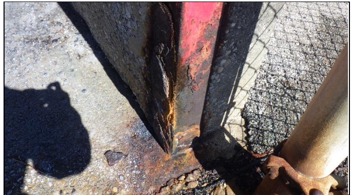
Gate corroding
