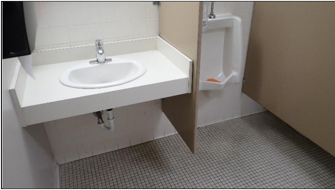
Overview of washrooms
