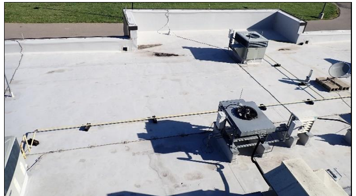
Overview of roof
