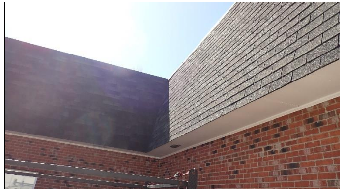
Overview of roof
