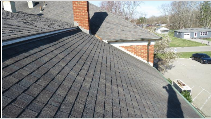
Overview of roof
