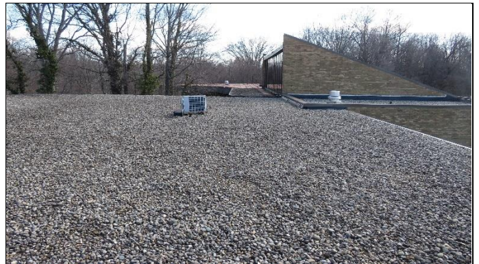
Overview of roof
