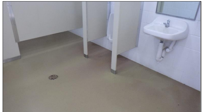
Overview of washrooms
