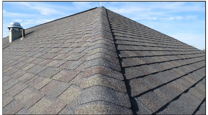
Overview of roof
