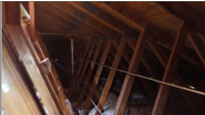
Overview of structure
