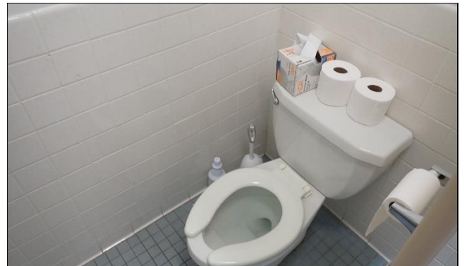
Overview of washrooms
