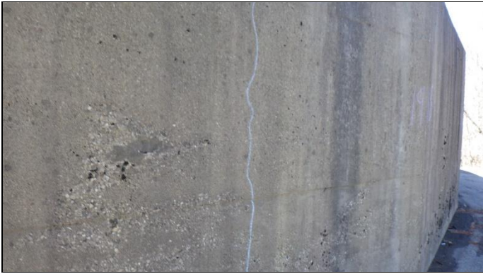
Foundation cracks
