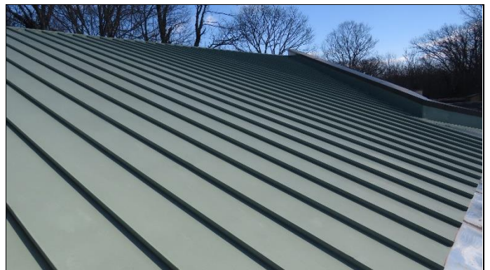
Overview of roof
