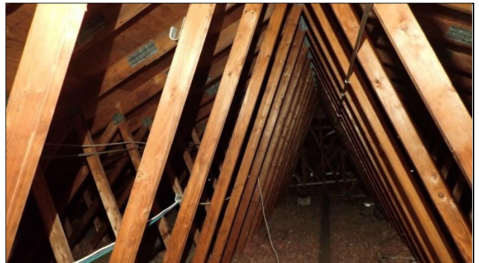
Overview of structure
