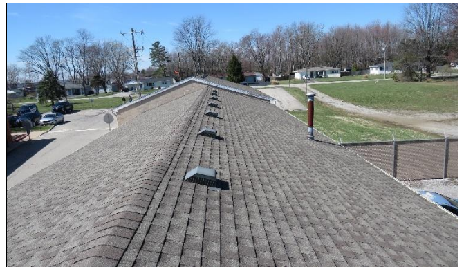
Overview of roof
