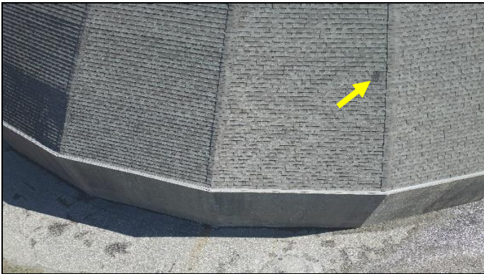
Displaced shingle
