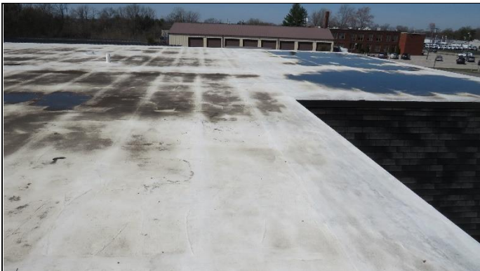
Overview of roof
