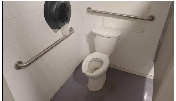
Overview of washrooms
