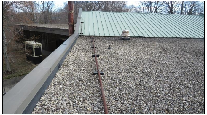
Overview of roof
