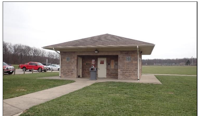
West washroom facility
