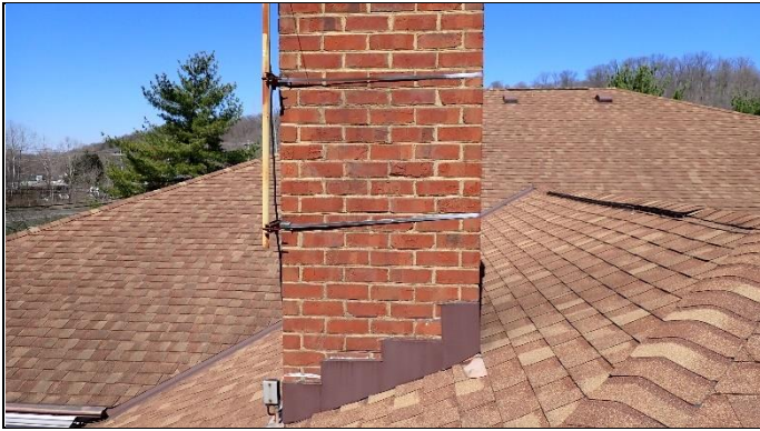
Overview of roof
