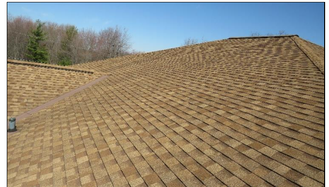
Overview of roof
