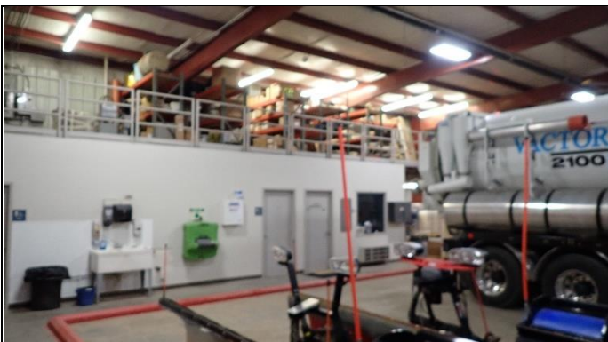
Overview of interior
