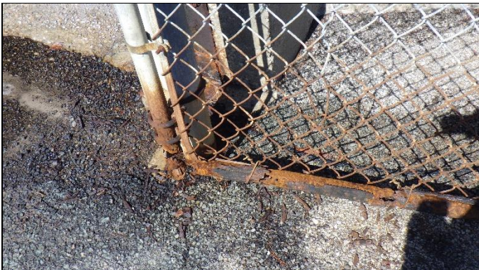
Gate corroding
