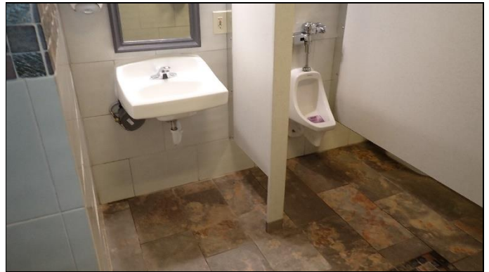
Overview of washrooms
