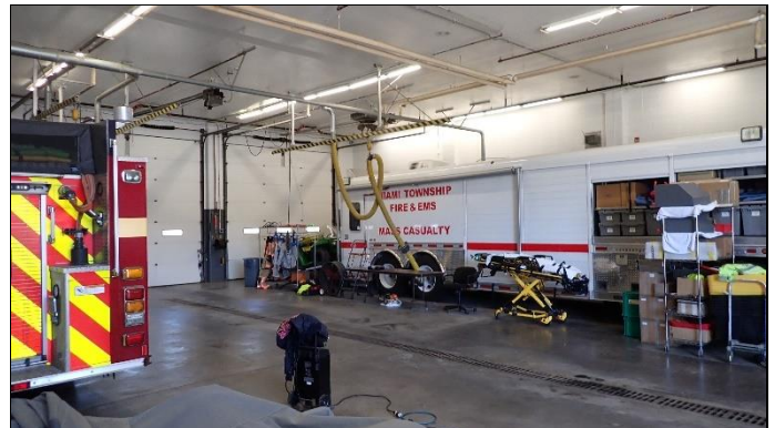
Overview of interior
