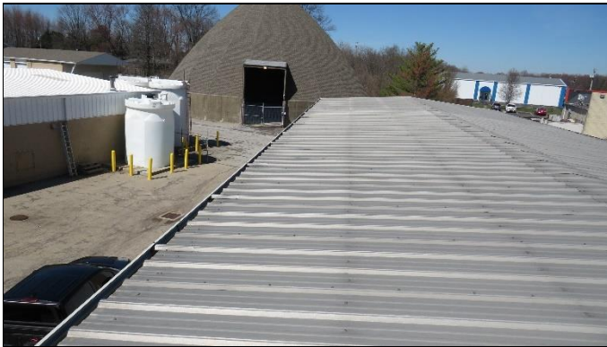
Overview of roof
