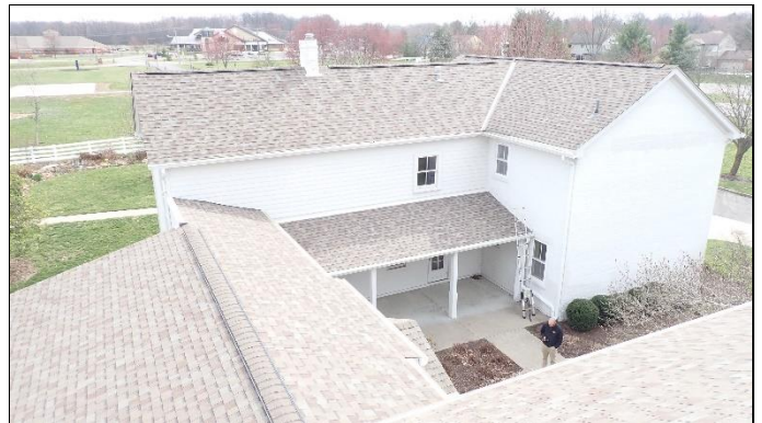
Community center roof
