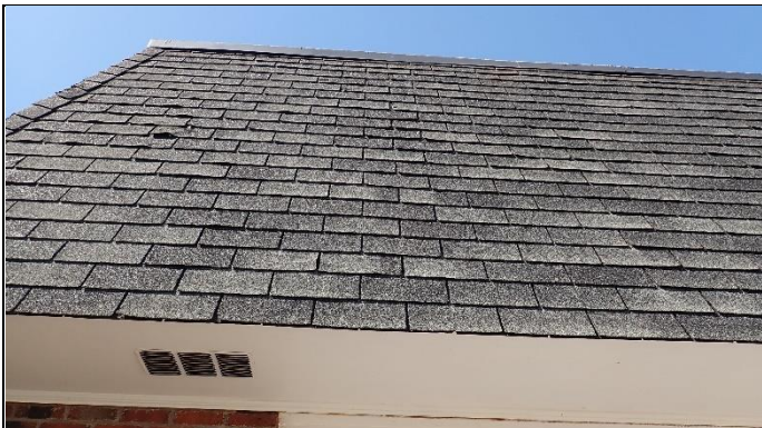
Overview of roof
