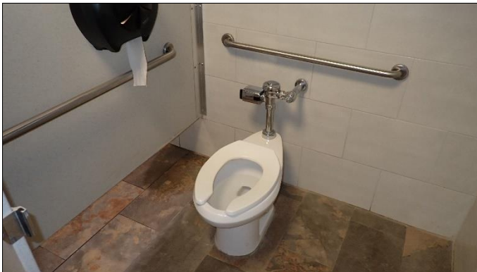
Overview of washrooms
