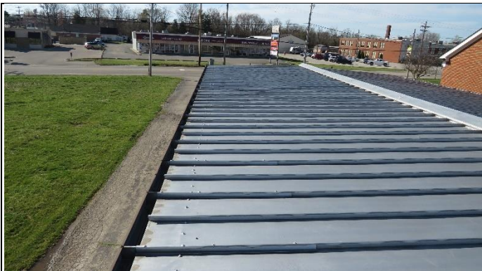
Overview of roof
