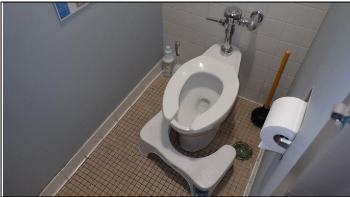
Overview of washrooms
