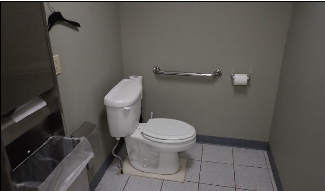
Overview of washrooms
