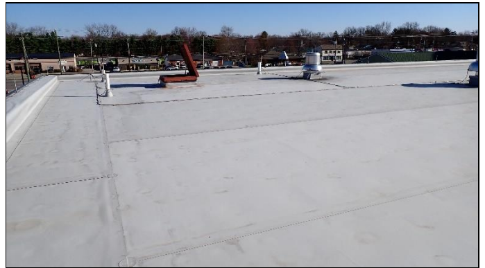
Overview of roof
