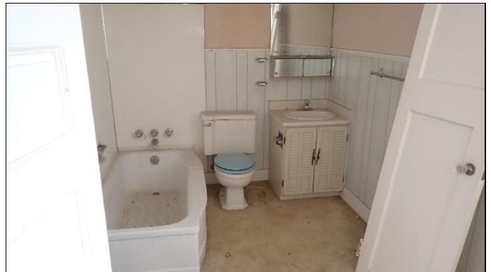
Overview of washrooms
