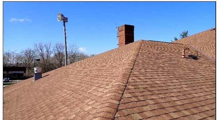
Overview of roof
