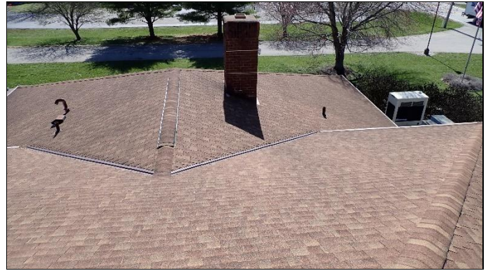
Overview of roof
