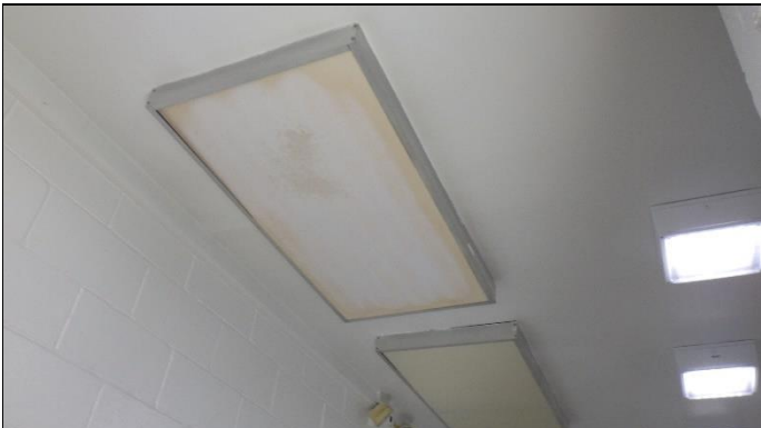
Overview of mechanical equipment
