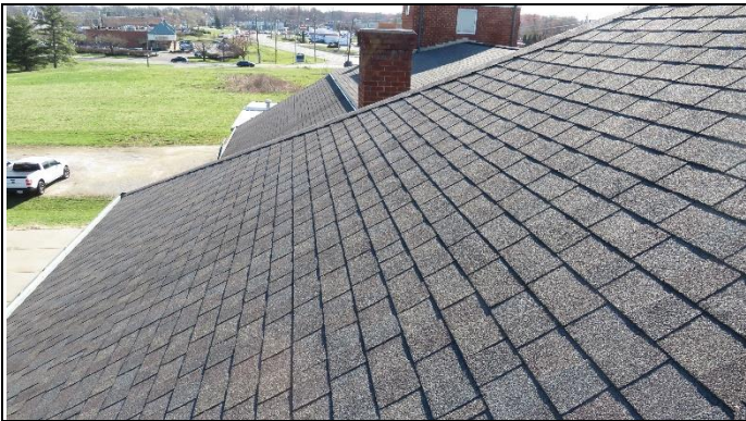
Overview of roof
