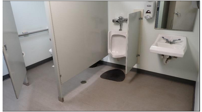
Overview of washrooms
