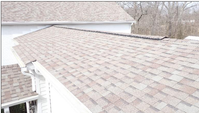
Community center roof
