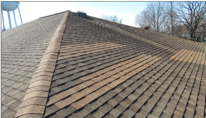
Overview of roof
