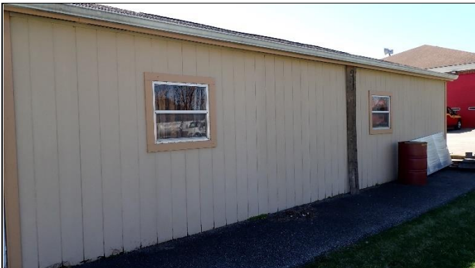
Overview of outbuilding
