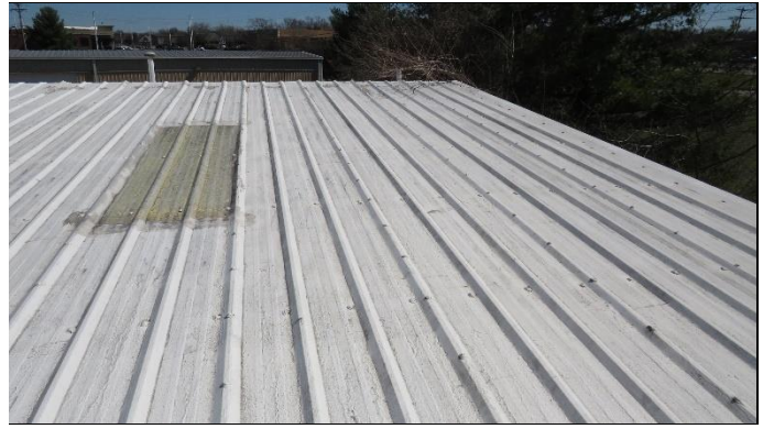
Overview of roof
