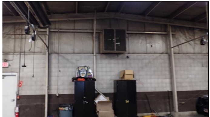
Overview of interior
