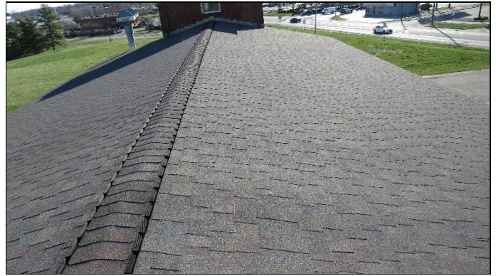
Overview of roof
