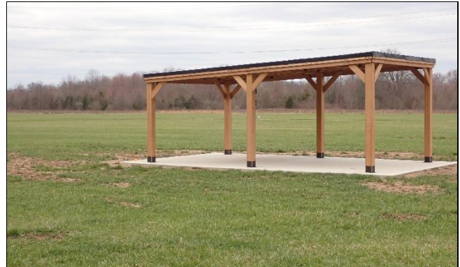
South picnic shelter
