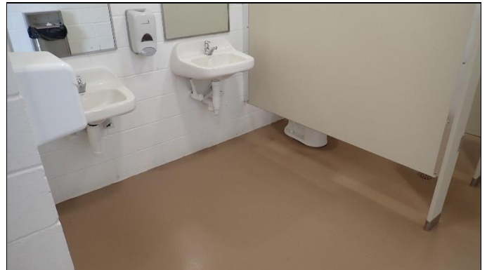
Overview of washrooms
