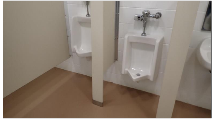
Overview of washrooms
