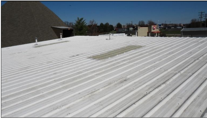
Overview of roof
