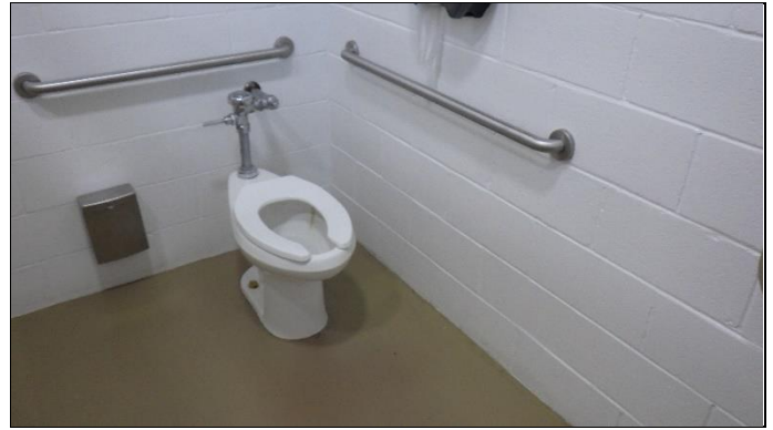
Overview of washrooms
