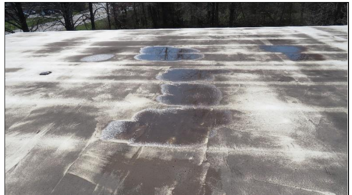
Overview of roof
