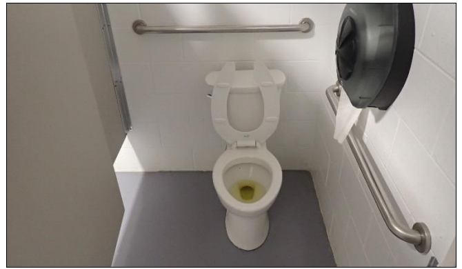
Overview of washrooms
