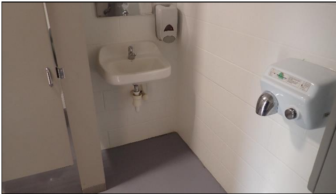
Overview of washrooms
