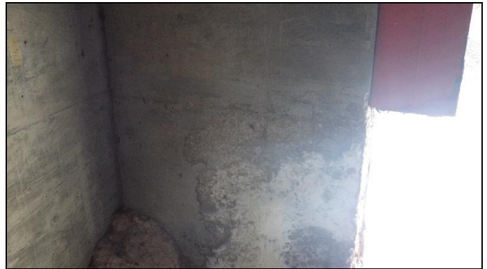
Concrete foundation wall
