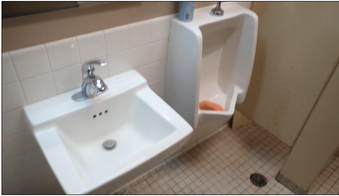
Overview of washrooms
