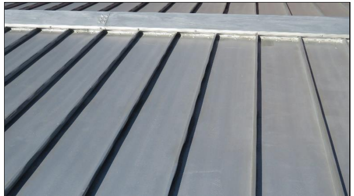
Overview of roof
