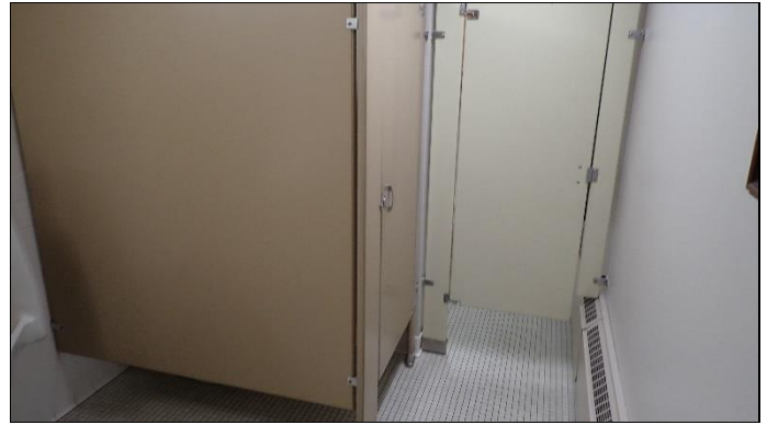
Overview of washrooms
