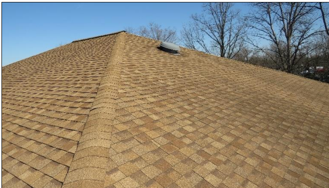
Overview of roof
