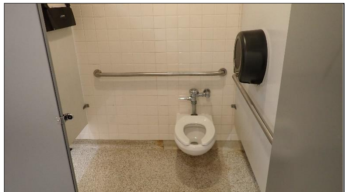
Overview of washrooms
