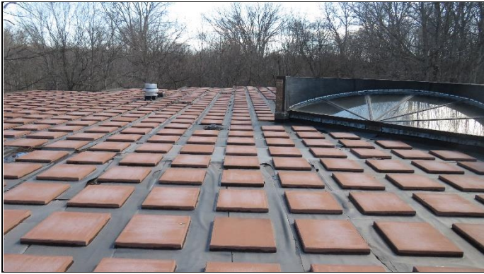
Overview of roof
