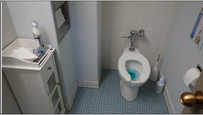
Overview of washrooms
