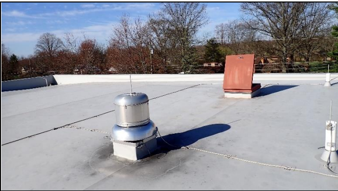
Overview of roof
