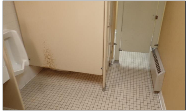
Overview of washrooms
