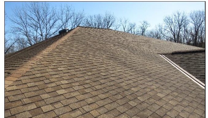
Overview of roof
