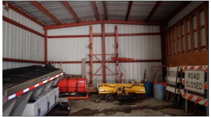
Overview of interior
