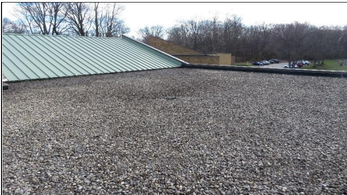
Overview of roof
