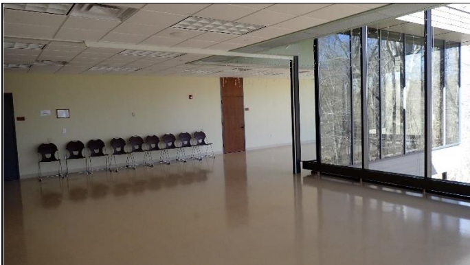
Overview of interior
