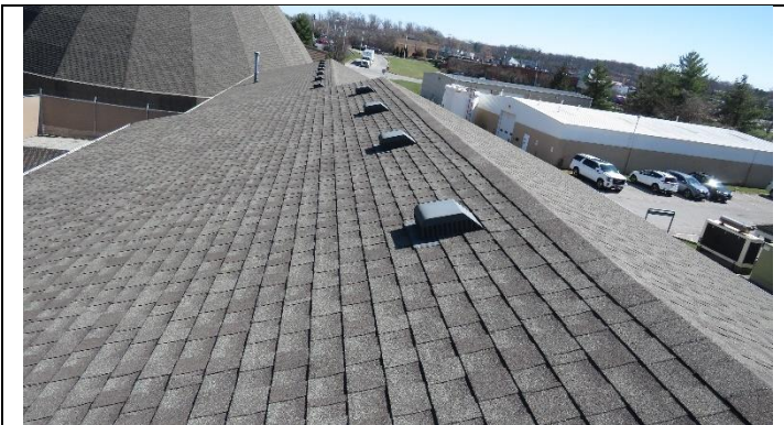
Overview of roof
