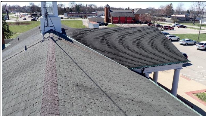
Overview of roof
