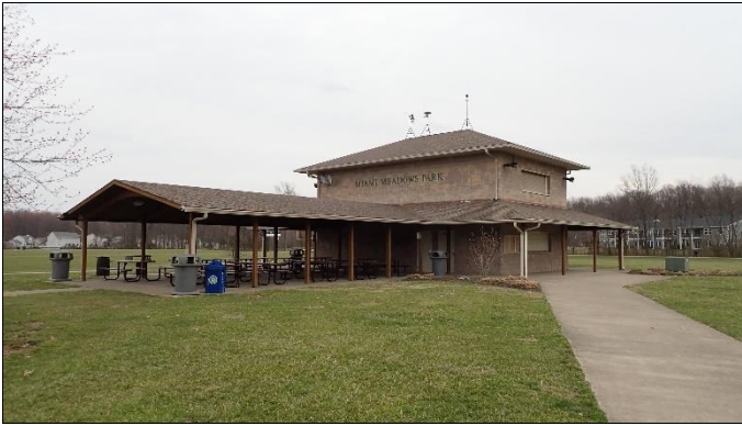
East concession and washroom facility
