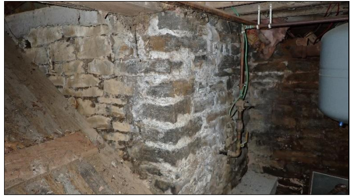
Overview of interior
