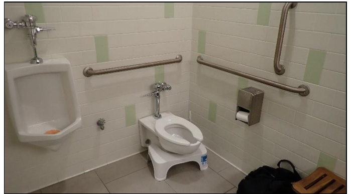
Overview of washrooms
