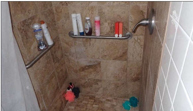
Overview of washrooms
