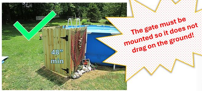
On a deck around an above ground pool, the fence and gate shall be at least 48" tall.
