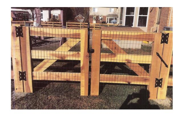
If the fence is open-face such as split-rail fencing, wire mesh is required on the outside of the fence.
