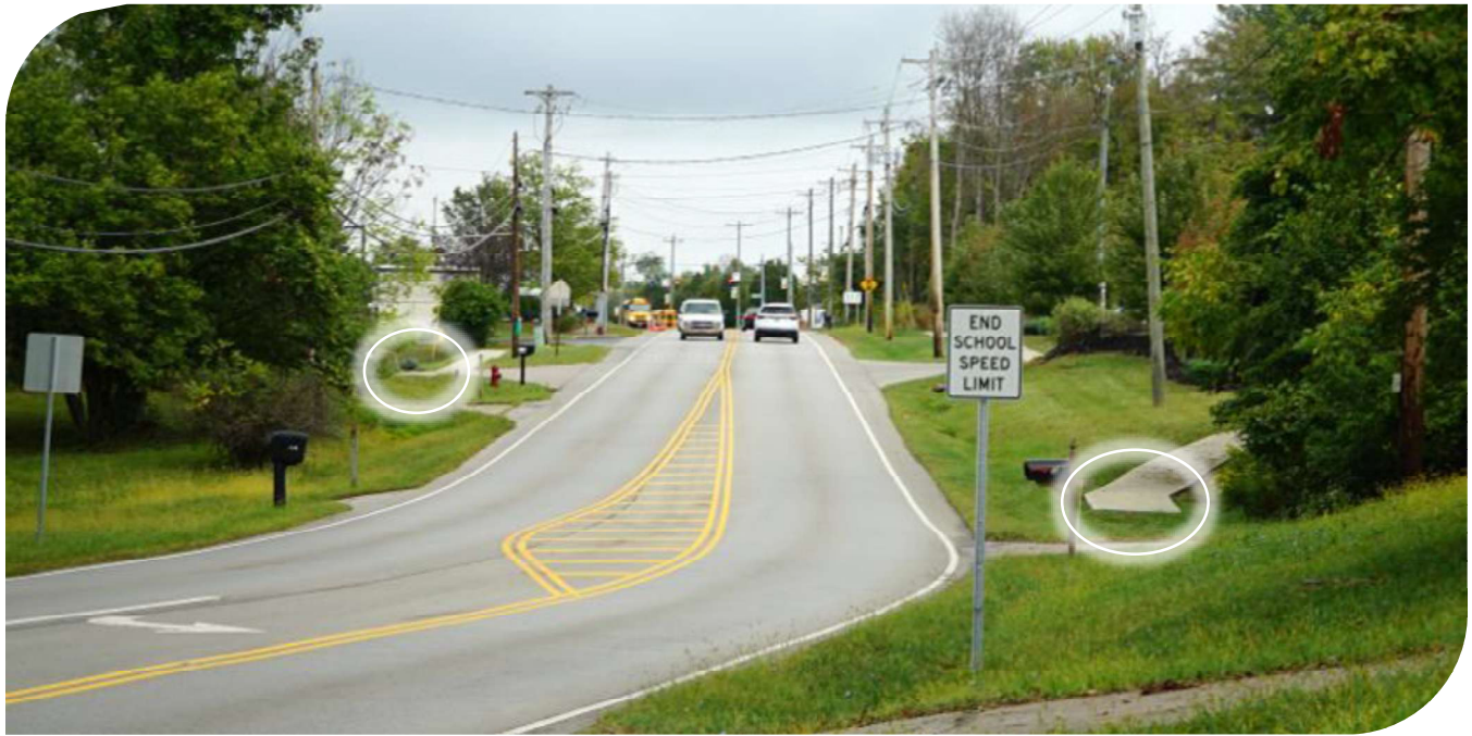
Figure 50. Sidewalk on Loveland-Miamiville Road terminates prior to reaching McCormick Elementary School
