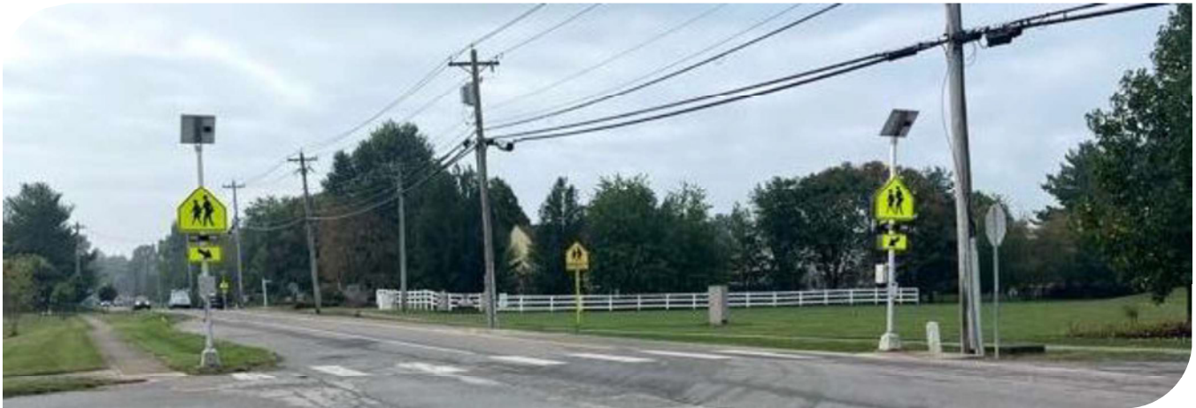
Figure 63. RRFB and high-visibility cross on Buckwheat Road at the school's south entrance
